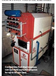
for the campus heating system. The Kohlbach product was selected due to its flexibility in handling a wide range of fuel moisture (up to 60 per cent) and variable sizes, coupled with the high quality of its design and manufacture. The system has a peak demand of 4.8MW, so the biomass boiler has been integrated with two 2.4MW gas fired boilers. The gasfired boilers top up output at peak times and offer full back up during maintenance periods.
